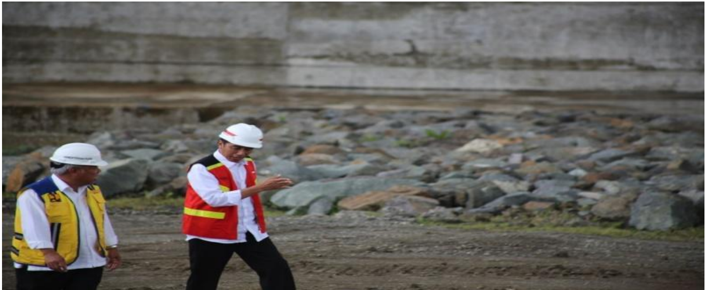
Figure 1: President of the Republic of Indonesia Ir. H. Joko Widodo accompanied by the Minister of Public Works and Public Housing, Dr. (HC) Ir. H. Mochamad Basoeki Hadimoeljono, M.Sc., Ph.D. while monitoring the construction of the Paselloreng Dam, Gilireng District, Wajo Regency, South Sulawesi. (Source: Personal Documents, 2018)
